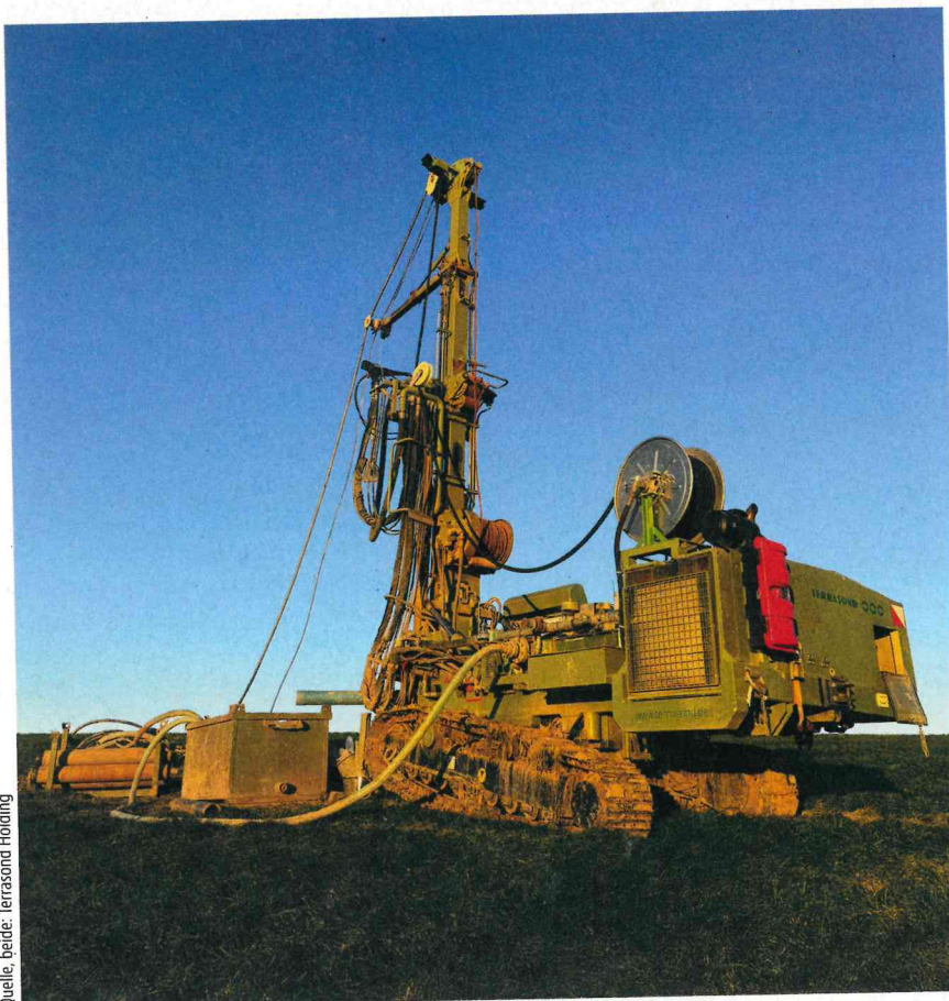
Quelle, beide: Terrasond Holding
